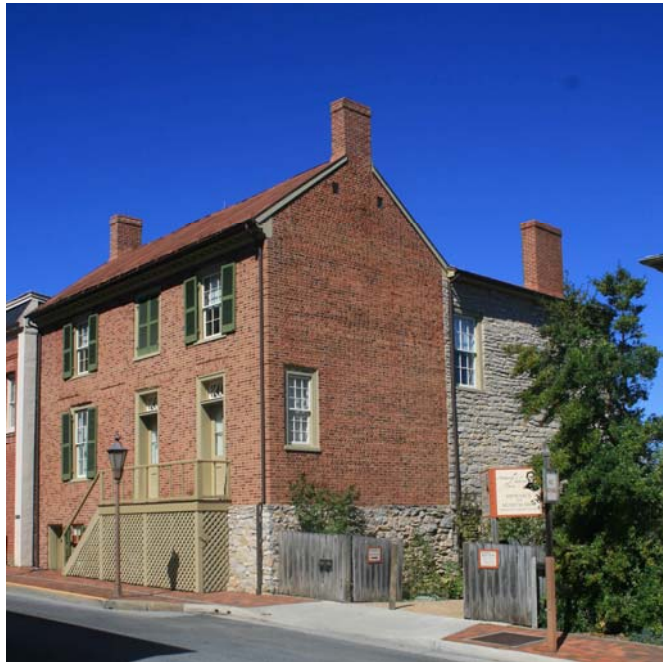
Stonewall Jackson House in Lexington. A joint proposal by the Stonewall Jackson Foundation and Virginia Military Institute would transfer ownership and operational responsibility to VMI.
